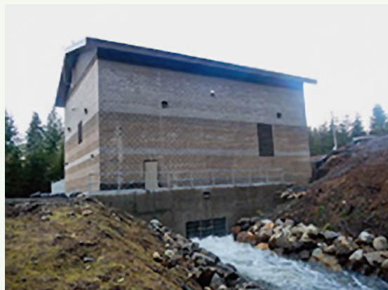
Calligan Creek Powerhouse (image courtesy of Snohomish PUD)
