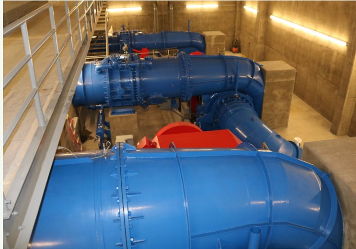
Pueblo Dam turbine-generator units (image courtesy of Kevin Meador, Southeastern Colorado Water Conservancy District)
